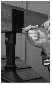
**10** Place the wood beam in the Saddle. Secure the beam with the 1/4" x 3" Simpson Strong-tie SDS structural screws (included). **Do not substitute fasteners!**  Sky
