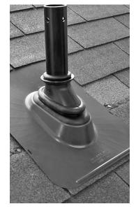
7 Install the pipe flashing by working the flexible boot over the Riser column. Follow manufacturer's instructions on securing the flashing to the roof. Reinstall the saved roofing material (removed in step #2) around the flashing.
