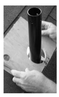
**5** Install backing and blocking under the edges of the opening. Use the saved plywood piece that was removed in step #3, then cut or drill a hole for the Riser. Secure the plywood piece to the blocking underneath.
