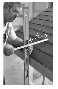
Determine approximate positioning of all SkyLift Riser brackets prior to cutting any access holes. The Risers must be positioned directly over exterior load bearing walls. Consider roofing layout, rafter locations, and interior conditions. Repositioning may be necessary due to discovered conditions.
